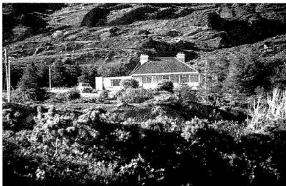
Figure 3. The cottage laboratory in Ireland.
