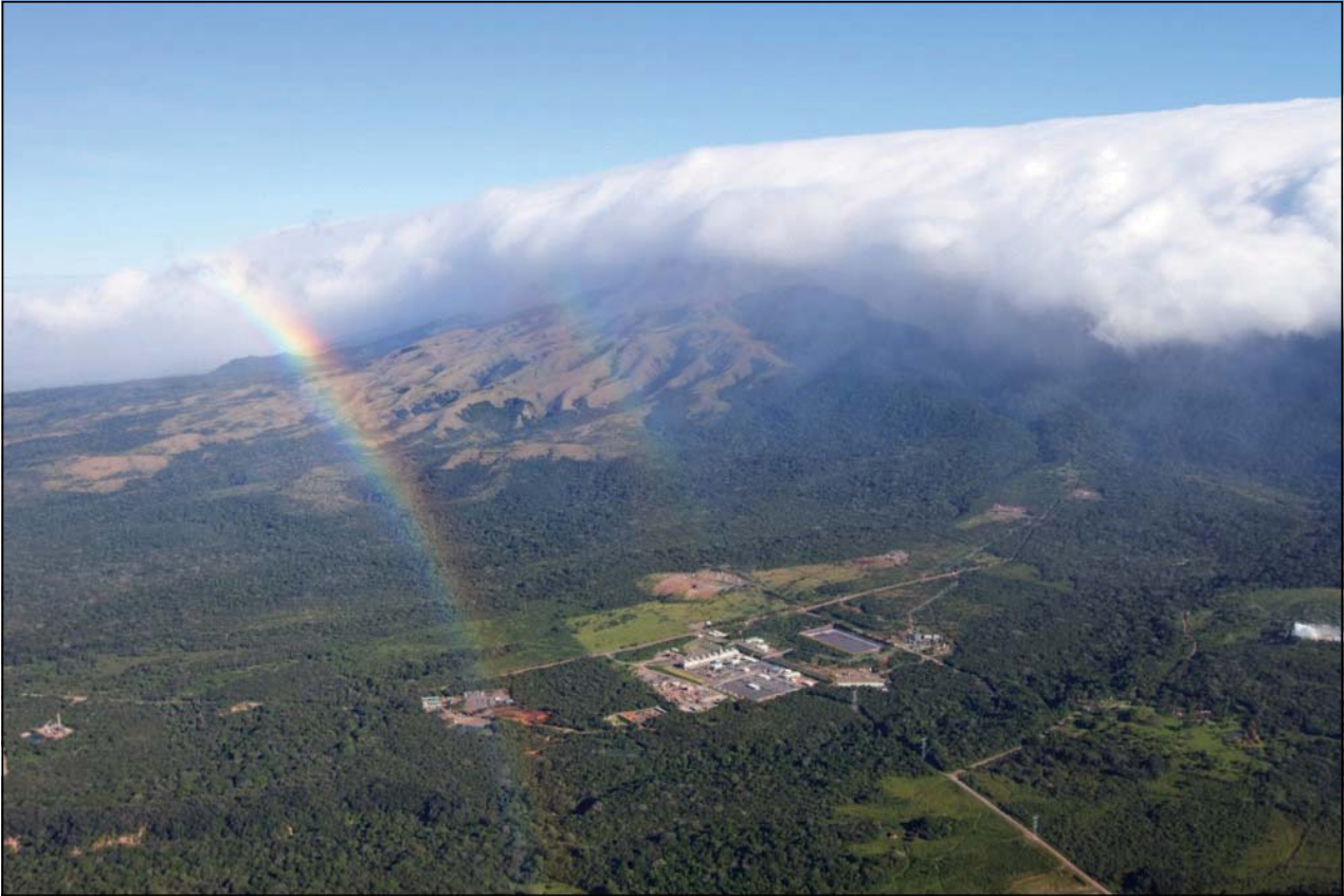
2011: Pailas Uno, geothermal power plant
