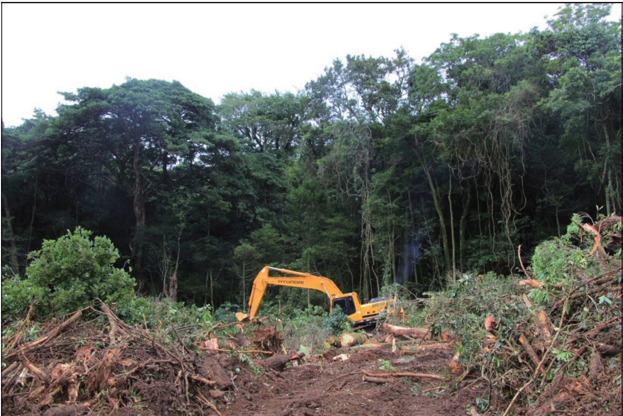
2013: clearing the forest
