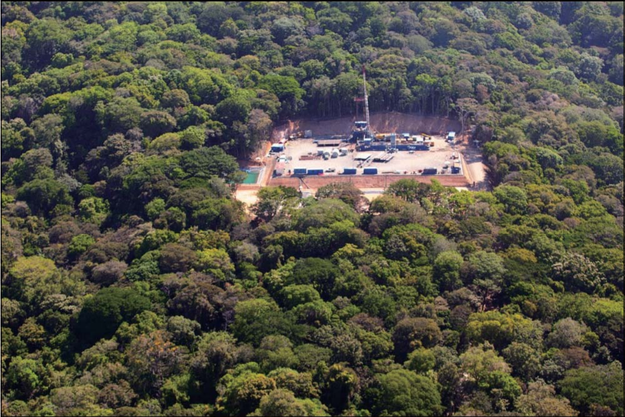
2013: the footprint, geothermal well
