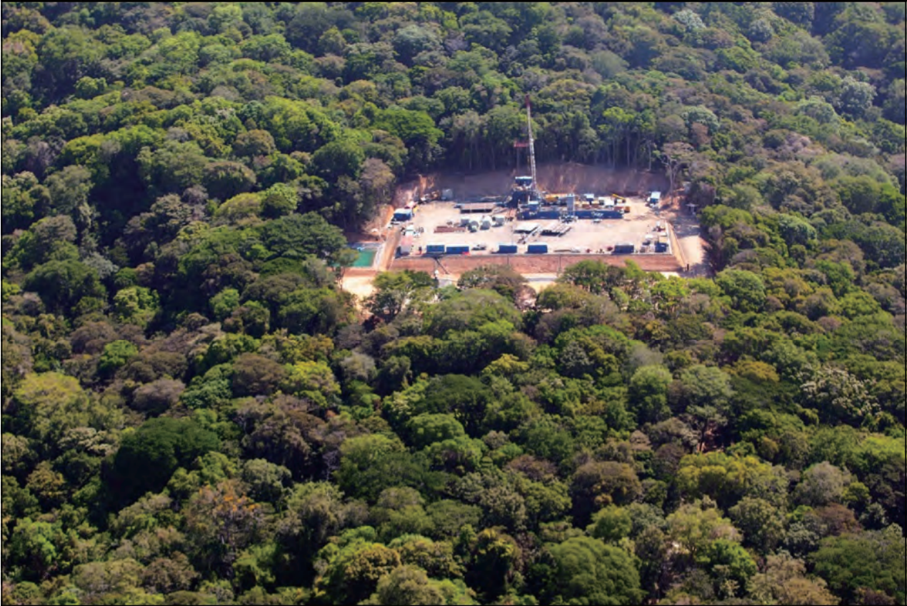
2013: the footprint, geothermal well
