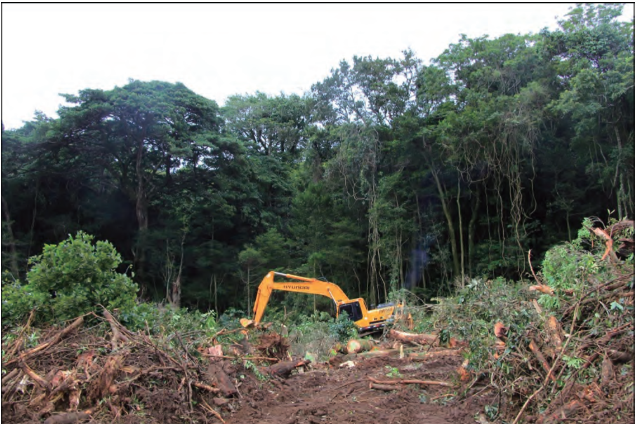
2013: clearing the forest
