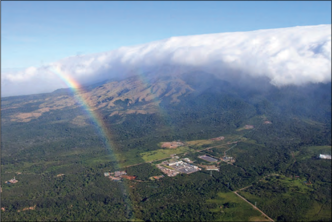
2011: Pailas Uno, geothermal power plant
