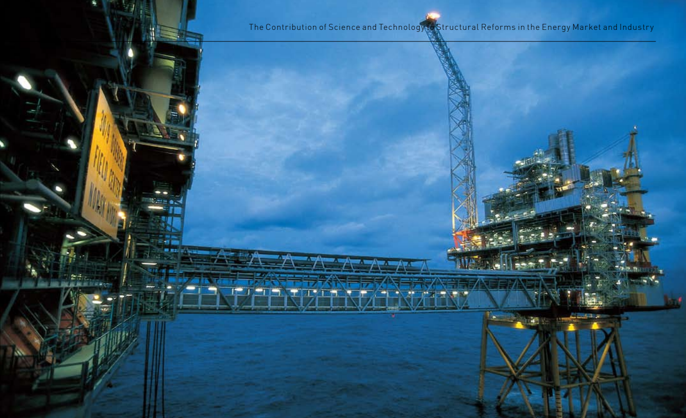
The Sleipner project implemented by Norwegian oil and gas companies in the North Sea Oil Fields is the world's first commercial carbon capture and storage project, where CO 2 contained in natural gas is captured and injected into saline aquifers 1,000 meters under the sea at a rate of 2,800 metric tons a day, using large marine equipment.
